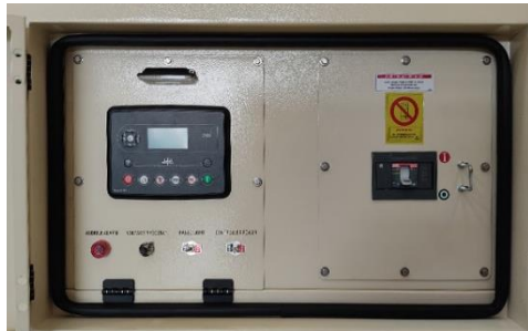
Control panel and breaker (rear side)
