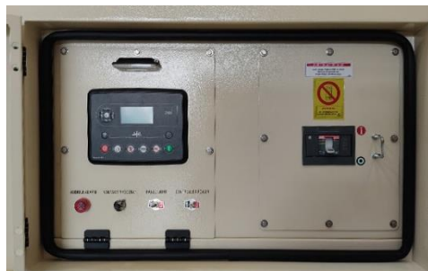
Control panel and breaker (rear side)
